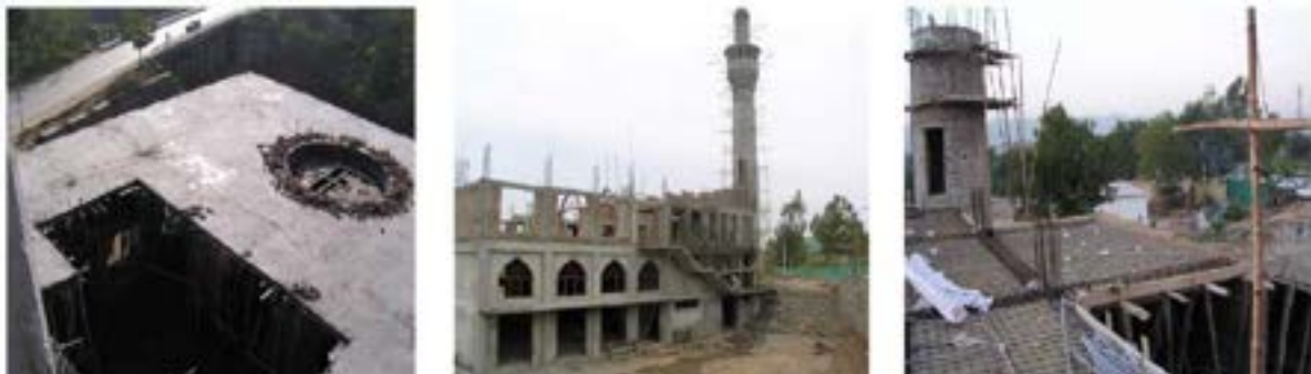
Construction Phases of the Mosque
