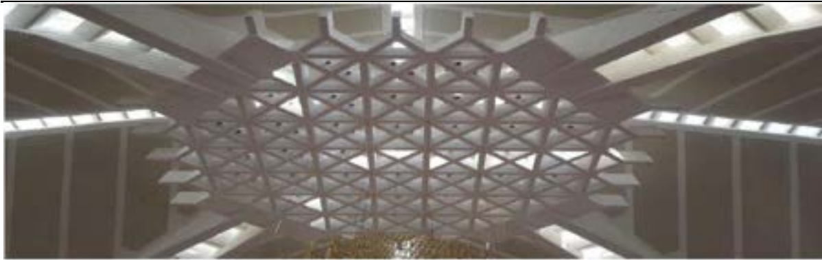
Roof design in main hall of Faisal mosque.
